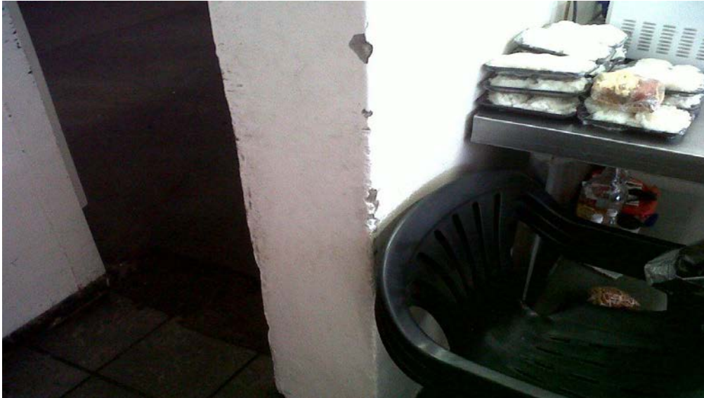
Photo 1 : Inspection of Food Premises for Compliance
